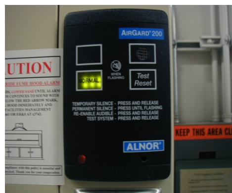
*Visible/audible alarm Sounds during low-flow condition
